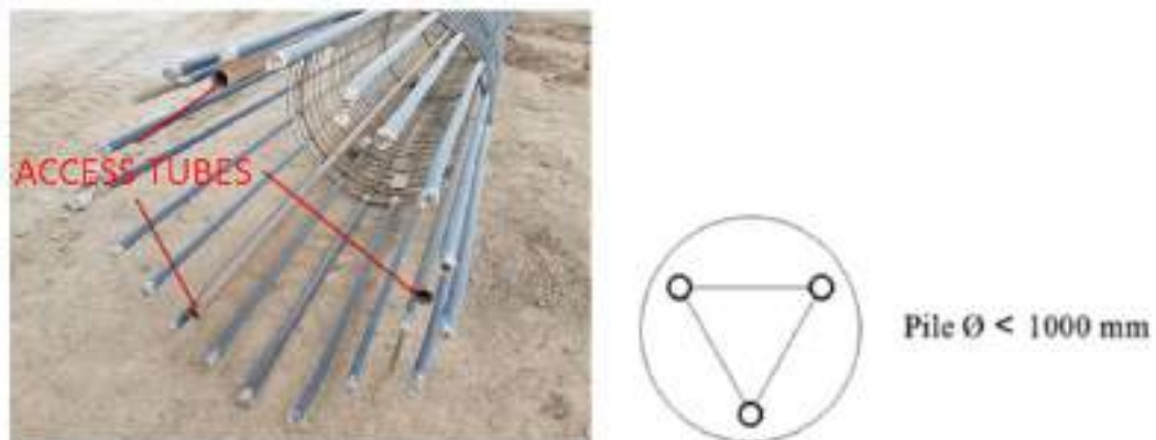
Figure 2 – Typical access tube configuration
